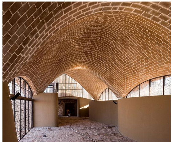
Figure 2. Mapungubwe interior vaulting 3
