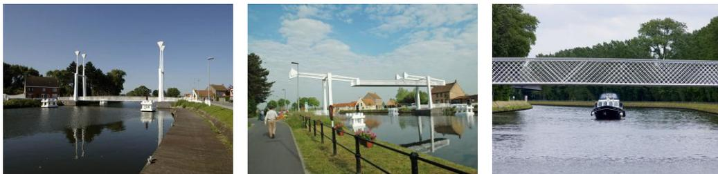
Figure 4. Footbridge Stalhille: Closed (left), Open (middle), and Close-up (right).<sup>10</sup>
